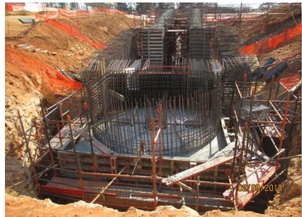
Construction of a sludge recycling pump station
