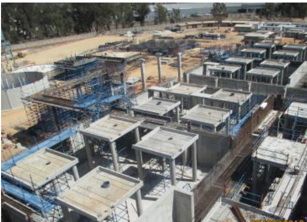
Construction of a reactor plant for pre-neutralisation and sludge-conditioning chambers
